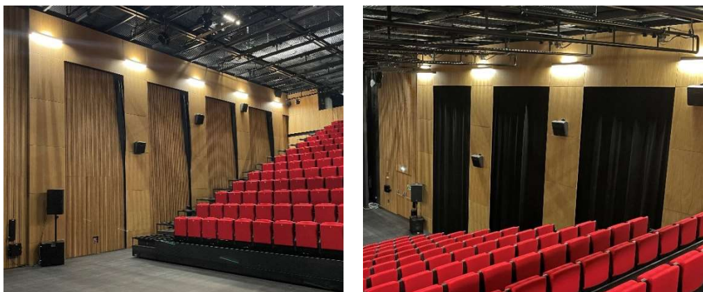
Figure 4 – Side wall diffuser panels without (left) and with curtains (right)
