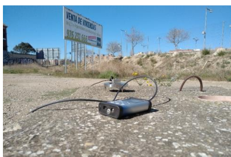
Figure 2 - Measuring the ground vibration in the site of the future building.
