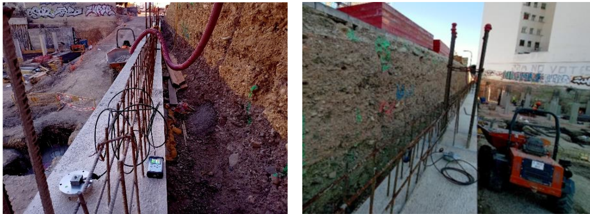
Figure 3 – Ground-borne vibration measurement at the foundation (at the pile heads).
