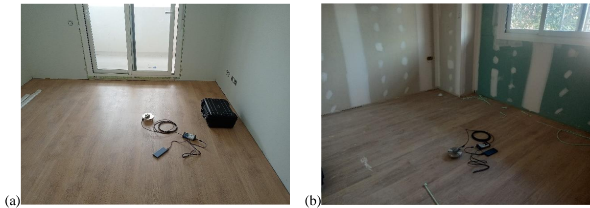
Figure 6 – The vibration measurement inside a closed space (a) above and (b) below the vibration cut.
